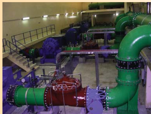
From left to right: Reservoir Data Monitoring Page and Abdaly Distribution Point
